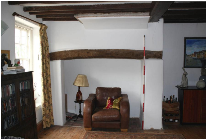
Figure 22. Inglenook fireplace and location of smoke hood in the south room (Dining Room). Facing southeast (IMG3581)
