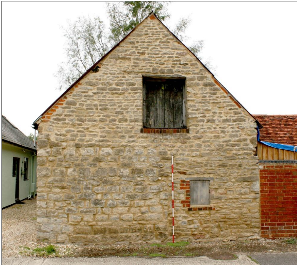
Figure 45. The carriage house. Southeast elevation with blocked entrance (IMG3685)
