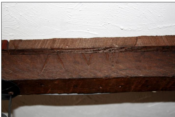
Figure 29. First floor. A to C: Carpenters marks on floor joists in the south bedroom (top: IMG3524; middle: IMG3526; bottom: IMG3525); D: metal bracket on joist in north bedroom
