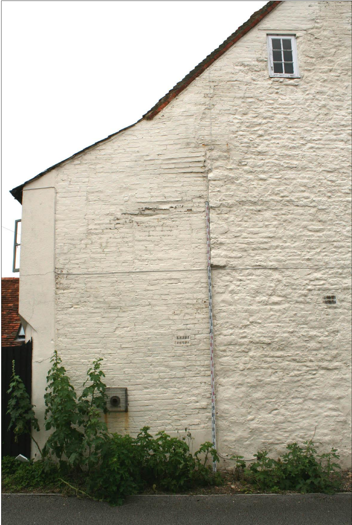
Figure 14. 19 th century extension. Southeast-facing elevation. Note: crude stretcher and stacked bond, and blocked window on first floor (IMG3689)
