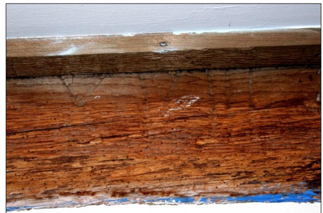
Figure 36. Second floor, south room partially concealed carpenter's numerals on southwest wall plate (IMG3483)
