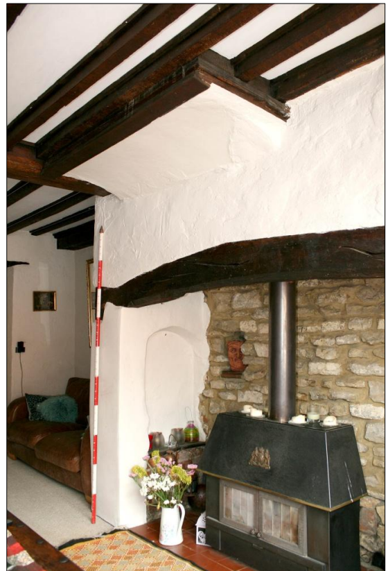
Figure 21. Inglenook fireplace in the north room (Living Room), showing location of smoke hood. Facing north west (IMG3564)
