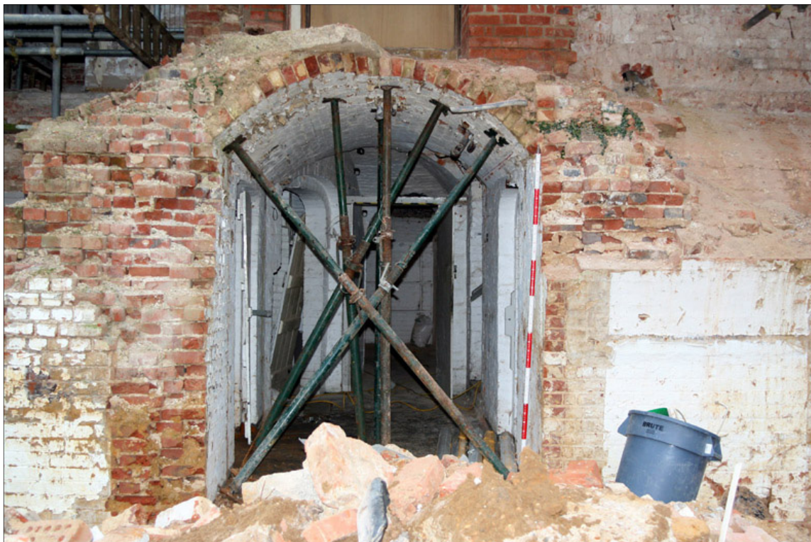
Fig.21. Viewpoint 15. Barrel vaulted corridor flanked by cells C (left) and D (right)
