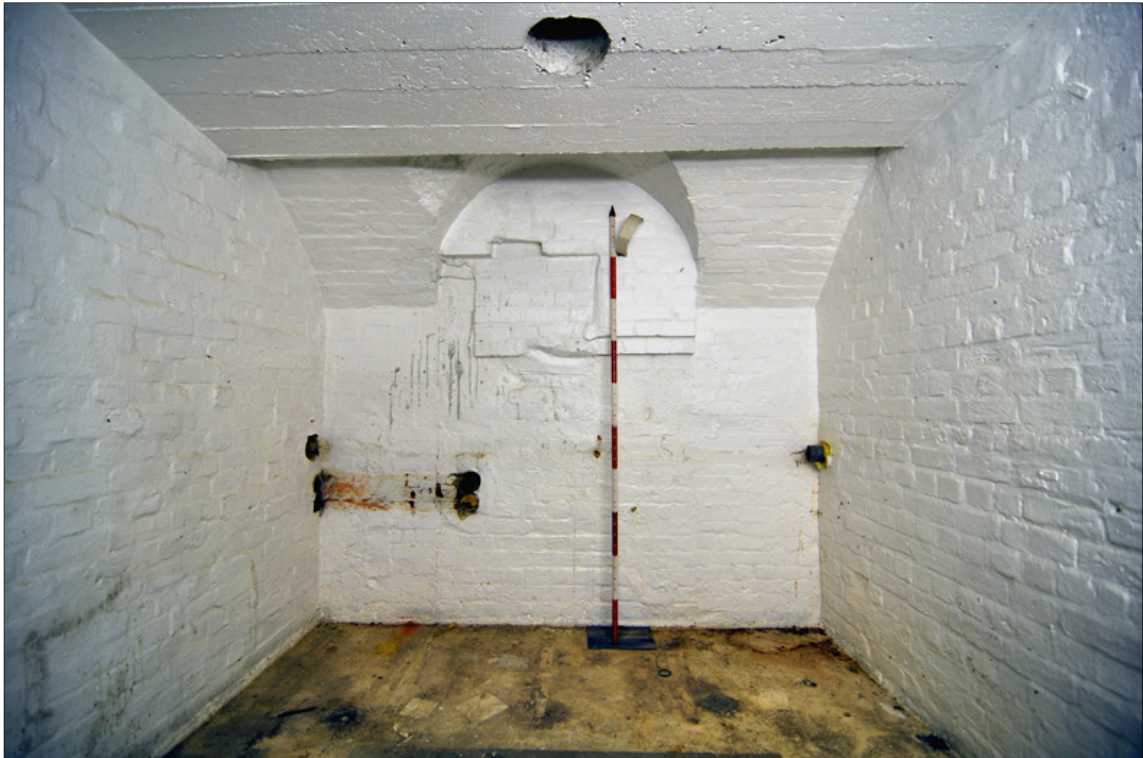
Fig.18. Viewpoint 12. Interior of cell B, showing blocked passage from cell A (secondary reinforcement partition walls to left and right)
