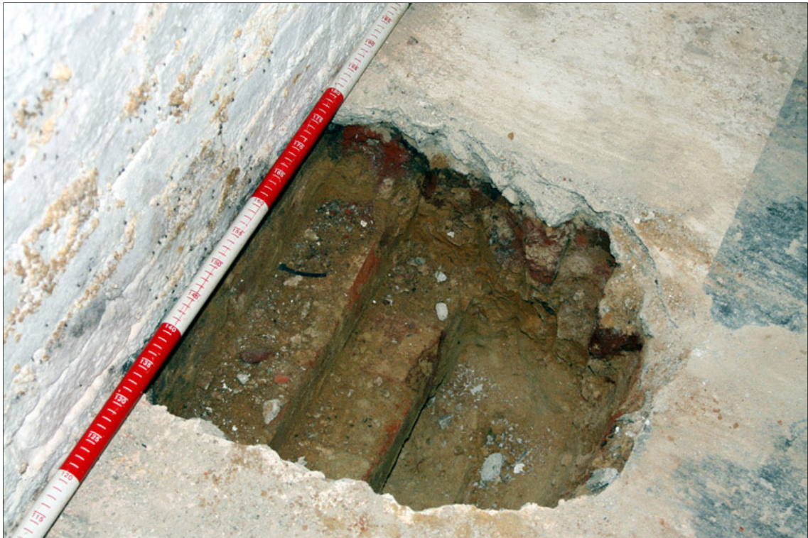
Fig.20. Viewpoint 14. Interior of cell B: exposed brick 'toe' foundation of north wall
